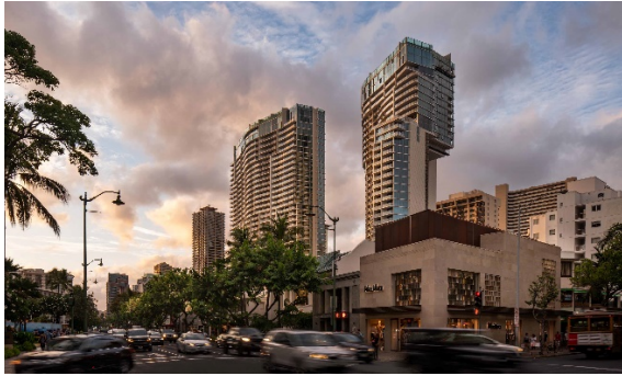
The twisting floor plan can be seen in this photo of the Phase 2 tower (right).
