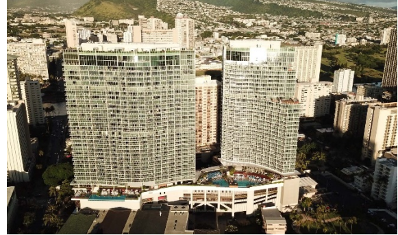
At right, the Phase 2 tower of The Ritz-Carlton Residences Waikiki Beach.
