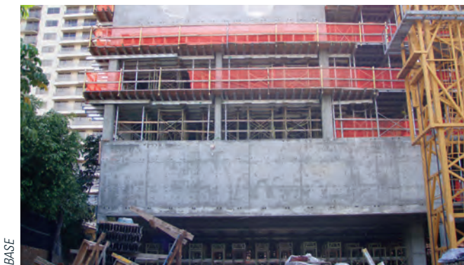
(left) Completed parking level transfer girders leveraged both upturned and downturned designs, depending on available space. (right) A 56-foot-long transfer girder on the second level was one of 23 required on the project.
