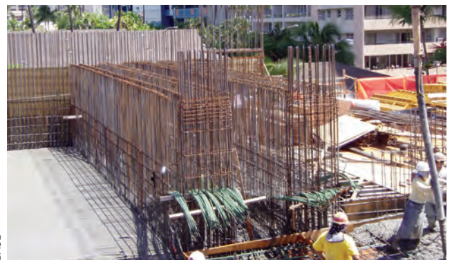
(left) Completed parking level transfer girders leveraged both upturned and downturned designs, depending on available space. (right) A 56-foot-long transfer girder on the second level was one of 23 required on the project.
