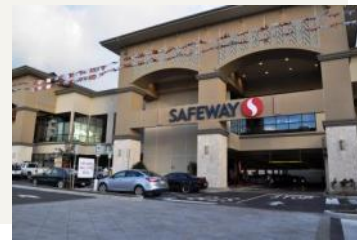
Safeway Beretania Contractor: Unlimited Builders, LLC Award of Excellence: Building Construction—$10-$25M General Contractors Association of Hawaii
