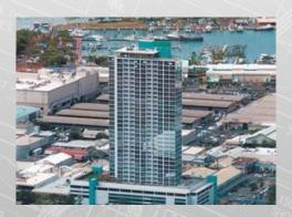
contractor for rapid estimating. The review also included optimizing the foundation, wall and slab design to achieve a potential \$2.1 million in savings. Additional benefits were achieved by eliminating dropped slabs in the tower allowing for more efficient and reduced cycle times for the forming systems.
