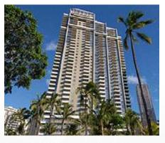
space. Value engineering identified \$1.3 million in potential savings and helped lead to a revised layout of the structure's lateral load resisting elements to increase the sellable floor area, providing the potential for an additional \$500,000 in sales revenue.
