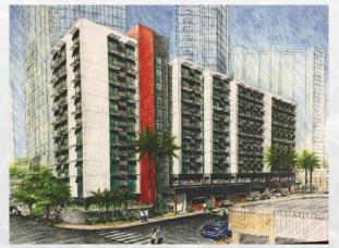
Construction is underway on this 11-story, 128-unit affordable rental project with a total height of 100 feet and approximately 153,000 GSF. Located on a constrained urban infill site the project had to incorporate parking and functional spaces under a residential tower of concrete tunnel-form construction.
