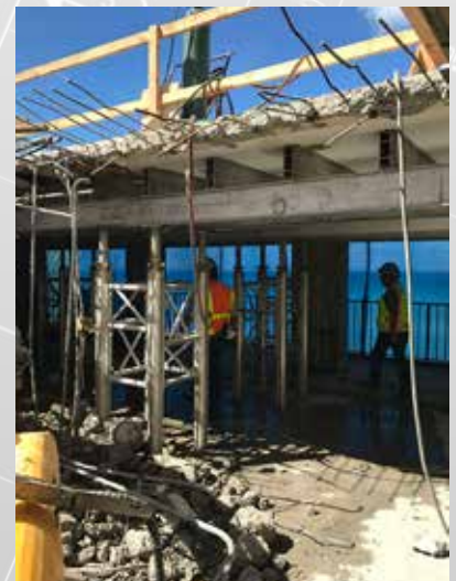
Shoring stabilizing remaining slab during reconfiguration of elevator and stairs cores.
