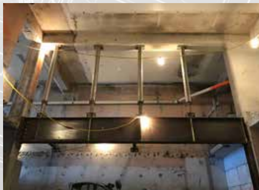
Transfer beam for shoring at ground floor to allow access for foundation installation.
