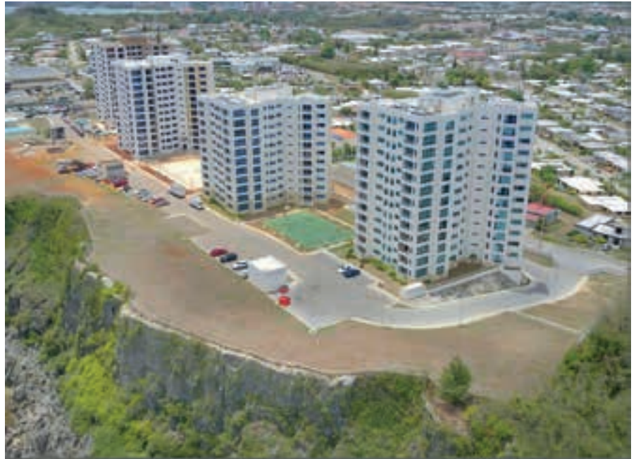
Summer Towers, a current Guam project by Core Tech International, a leading Pacific Region GC PHOTO COURTESY CORE TECH INTERNATIONAL
