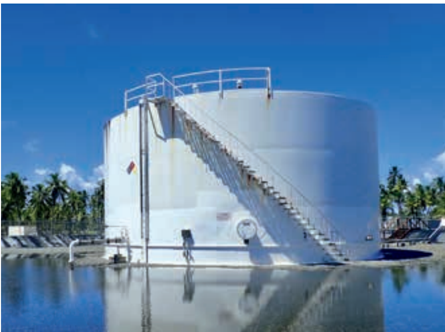
Nan Inc. will repair Fuel Tank #2 on Roi Namur, RMI PHOTO COURTESY NAN INC.
