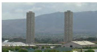
Fig. 1—Century Park Plaza Towers.
