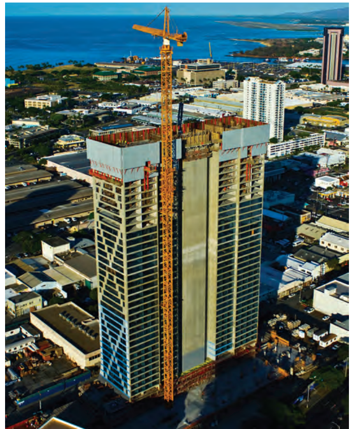
Fig. 2—Pacifica Honolulu under construction.
